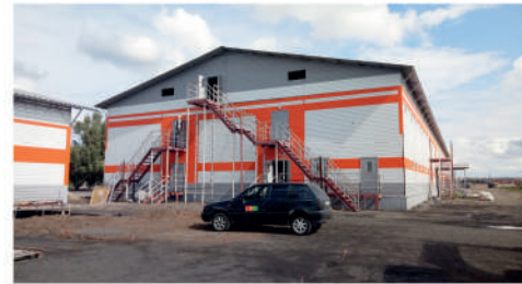
Modular building of a shower complex for 1,600 persons
