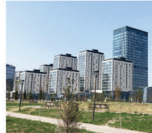
Green Block Residential Complex
